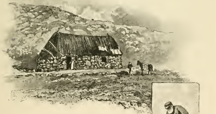
DRYING TWEED ON ROOF OF HOUSE.
